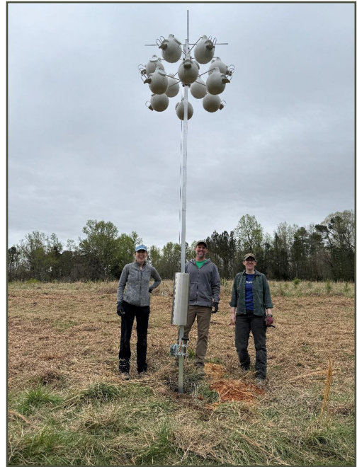
Gourd house installation at Blackwood Farm Park. Photo by Barbara Driscoll
